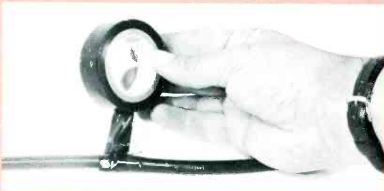
(D) Tape joint with good-quality electrical tape.
